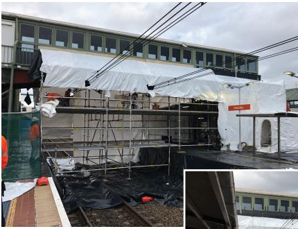
The scaffold is covered in a high-grade polymer and heated to form the encapsulation. This process provides safe containment of hazardous particles during the removal process.
