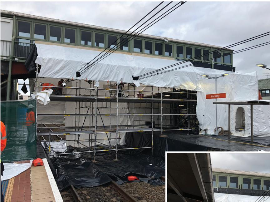
The scaffold is covered in a high-grade polymer and heated to form the encapsulation. This process provides safe containment of hazardous particles during the removal process.
